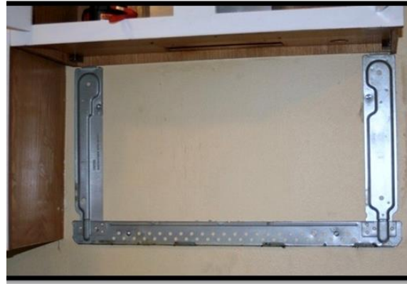
Mounting bracket secured and installed
