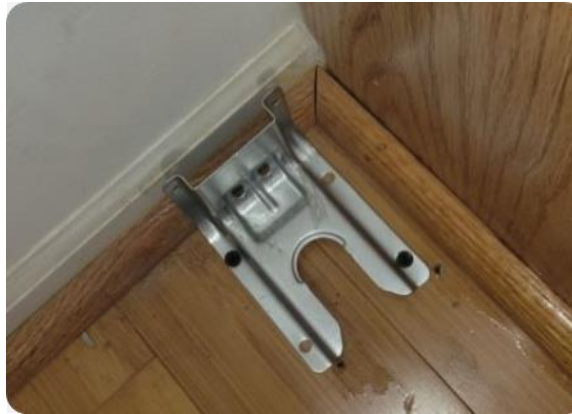
Document Anti-tip Device installed
