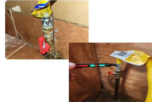
Illustrate connections have been made and tested for leaks.
