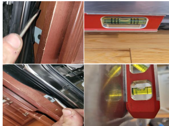
Illustrate how you've mounted & leveled the unit, causing no damage to cabinetry. Cabinetry claims are the #1 reason for claims with built-in appliances. Unlevel units are the #1 reason for service calls.
