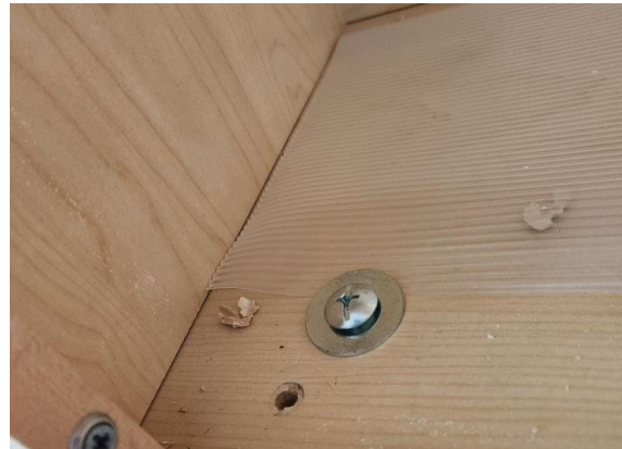
Mounting bolt flush with cabinetry
