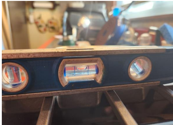
Ensure unit is level to meet manufacturer specifications
